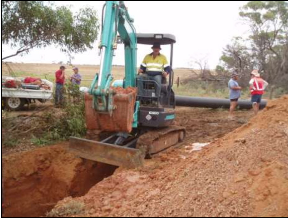
Fig 42: The local landholders discussing the new drain
