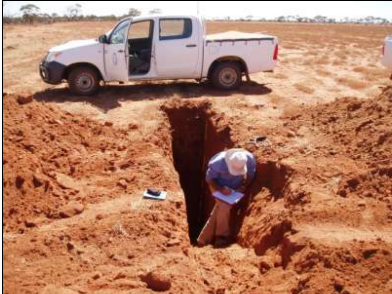
Fig 8: Carrying out soil sampling in a backhoe pit, Canna Gutha
