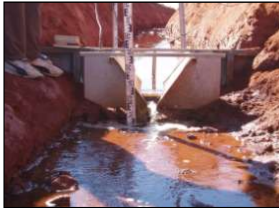
Fig 22b The finished flume
