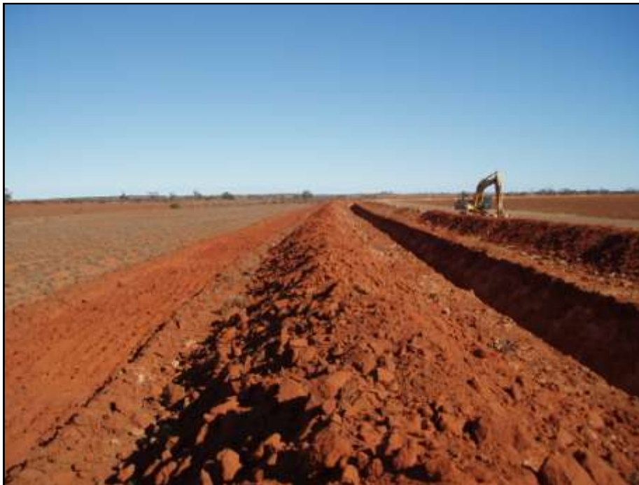
Fig 17: Taken at Canna Gutha. Surface water channels either side of the levee banks flanking the central deep groundwater drain.
