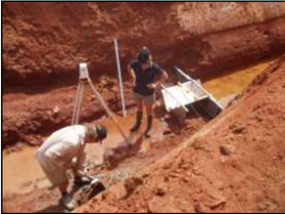
Fig 22a Constructing the flume at Merkanooka
