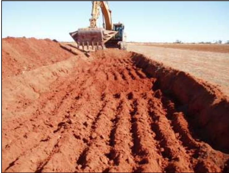
Fig 18: Construction of the surface drain, taken at Canna Gutha
