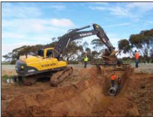
Fig 53: Installing the under rail crossing at Burakin
