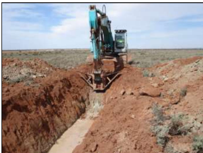
Fig 50: Excavation in Mongers 16
