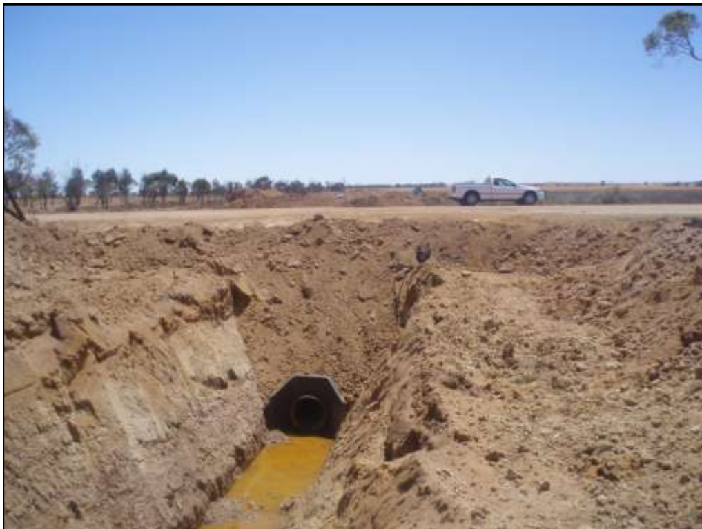
Fig 43: Wasley Road culvert
