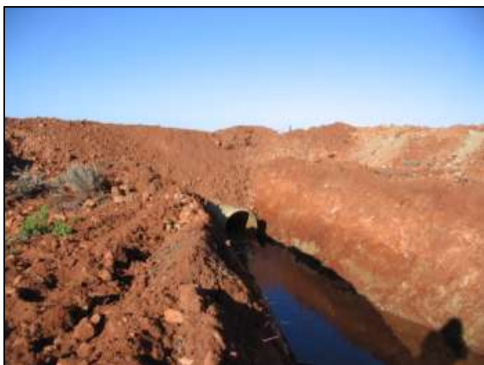
Fig 51: Culvert under Simpson Road, Mongers 16
