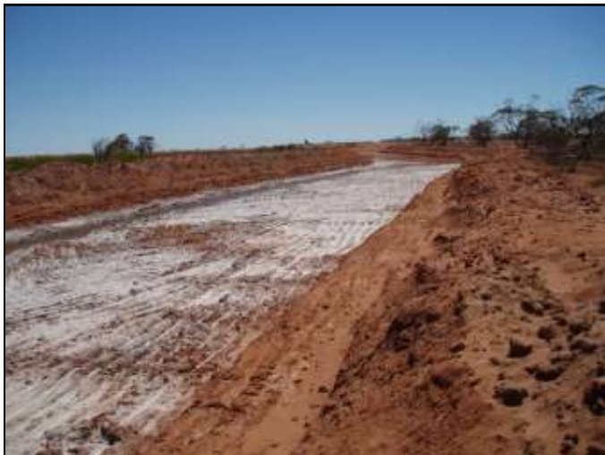
Fig 37: The Merkanooka surface water channel following de-silt.
