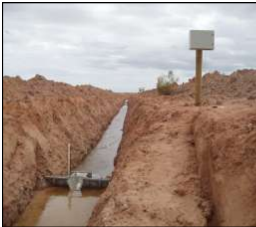
Fig 23a: Jibberding flume and monitoring station
